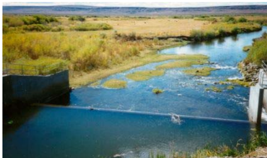
Figure 44. Duck Valley's new and improved water system.
